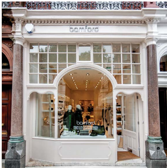
Façade, 62 South Audley Street
